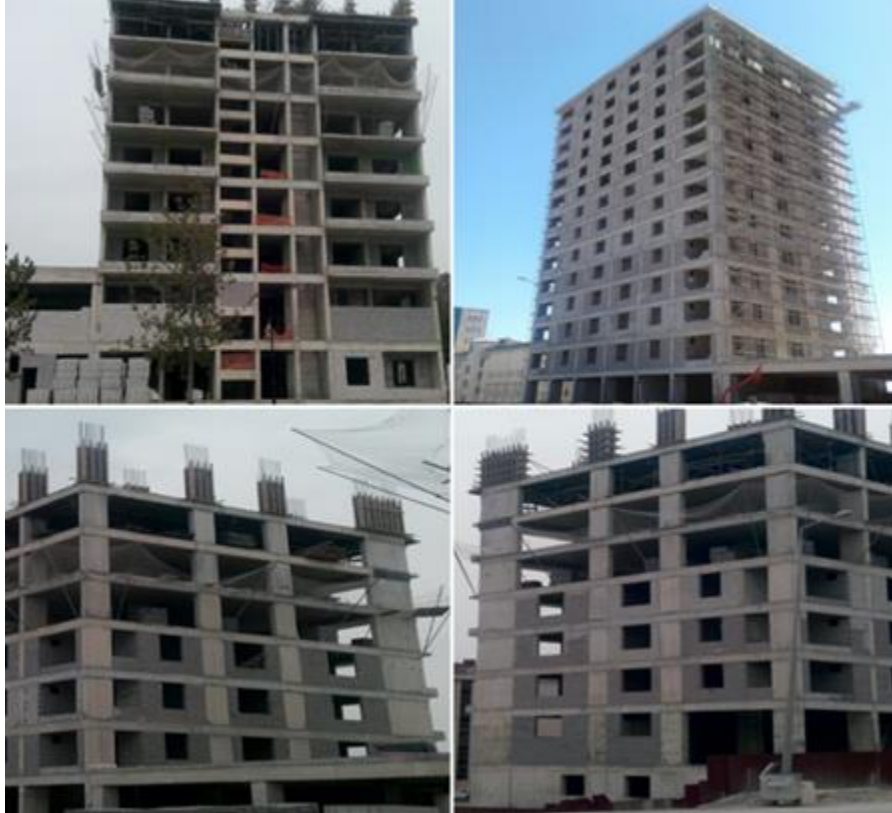
Figure 9. Various views of the application building with the Shear Wall-Frame carrier system during the construction phase
